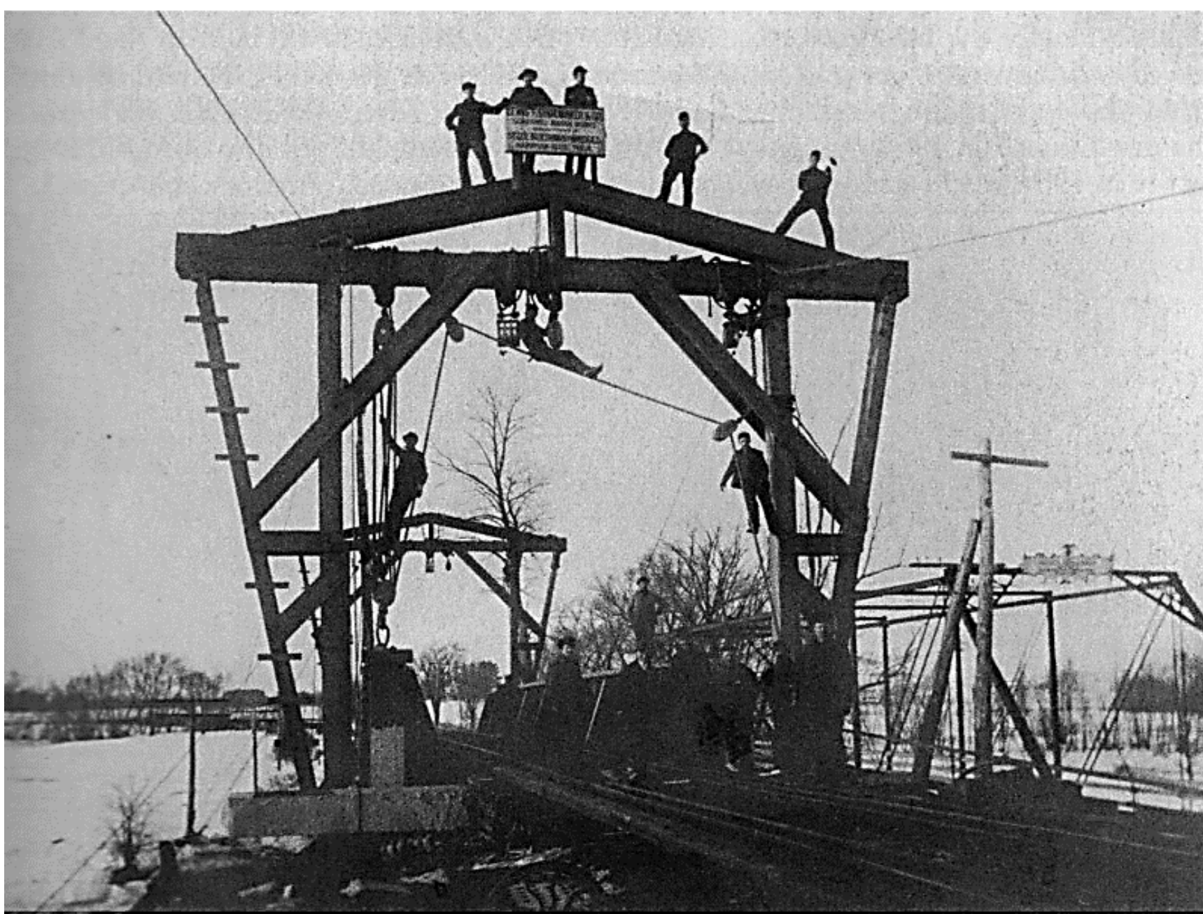
Building the Ashley Falls Railroad Bridge
