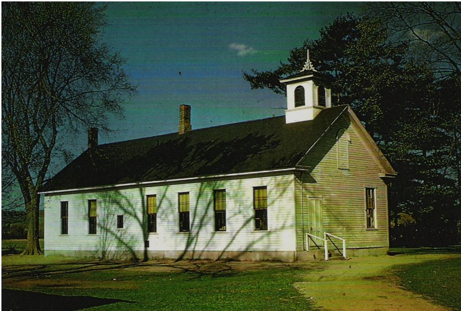
Community Center On Clayton Road near the cemetery.
